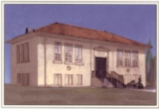
CARNEGIE TECHNOLOGY CENTER
