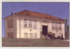
CARNEGIE TECHNOLOGY CENTER
